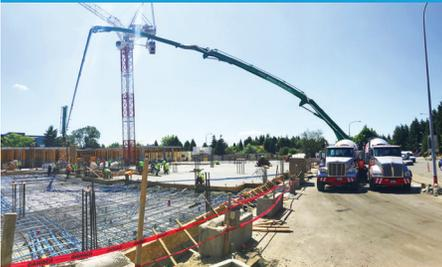
**When NITROcrete was added to their process, not only did Best-Way minimize cost and risk, but they also consistently cooled the 90-degree concrete to 50-degree batches.**
